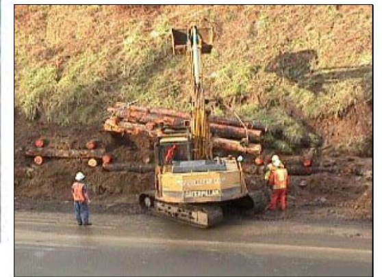
Live cribwall during construction. USDA Forest Service
