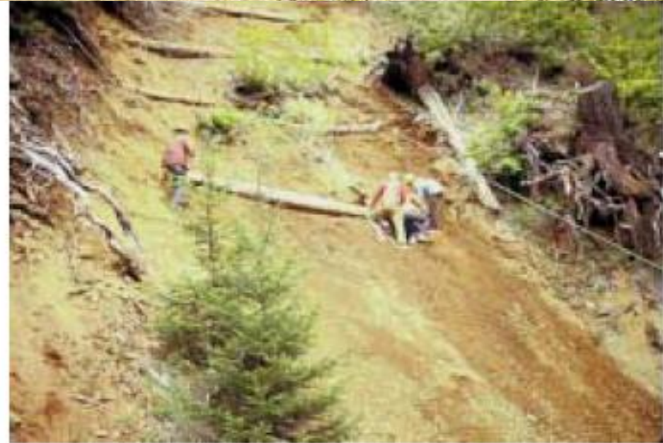
Installation - cutslope stabilization with log terracing. USDA Forest Service
