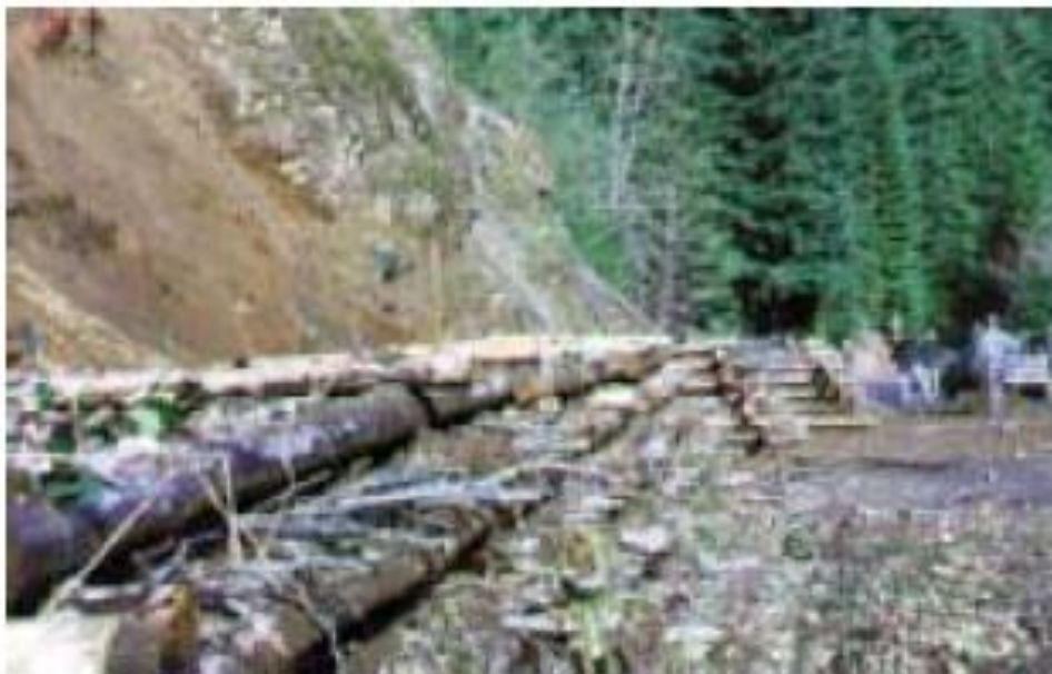
Live cribwall during construction. USDA Forest Service
